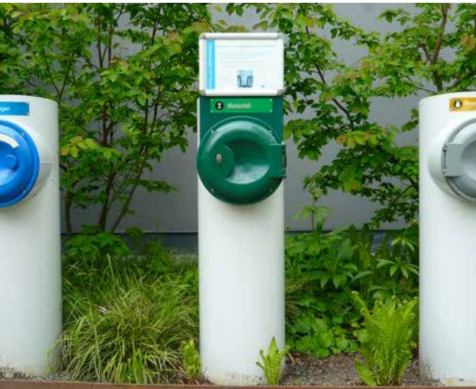
Figure 4.3.1b - Vacuum waste collection technologies
