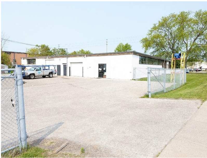
Image 15: View of 1072 and 1076 Rangeview Road.
