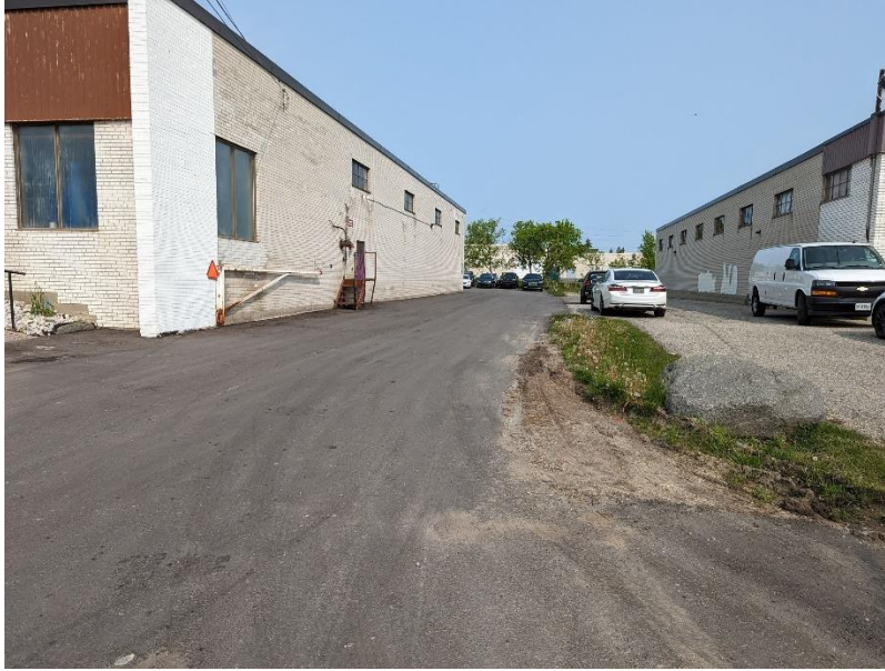
Image 21: View of 1025 and 1035 Rangeview Road.
