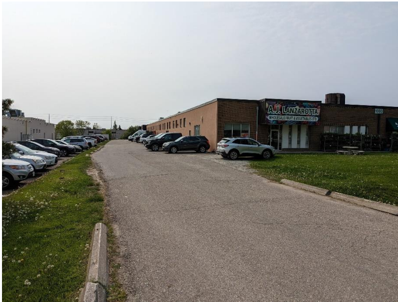
Image 12: View of 1050 Lakeshore Road East.
